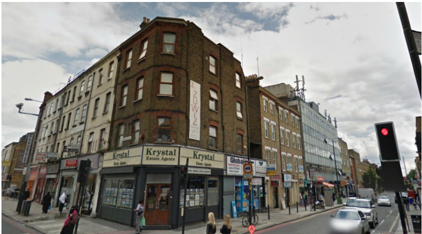
It used to be called Frumkins Corner.. 162 Commercial Road in the 21st Century
